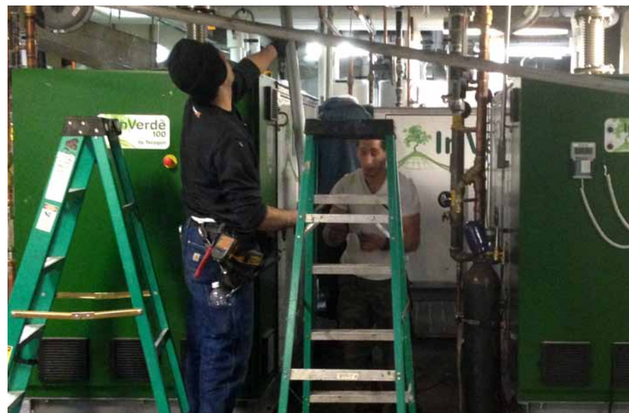
Workers finalize the installation of a new 300-kilowatt combined heat and power plant that will efficiently supply electricity and domestic hot water to a New York City housing complex.
