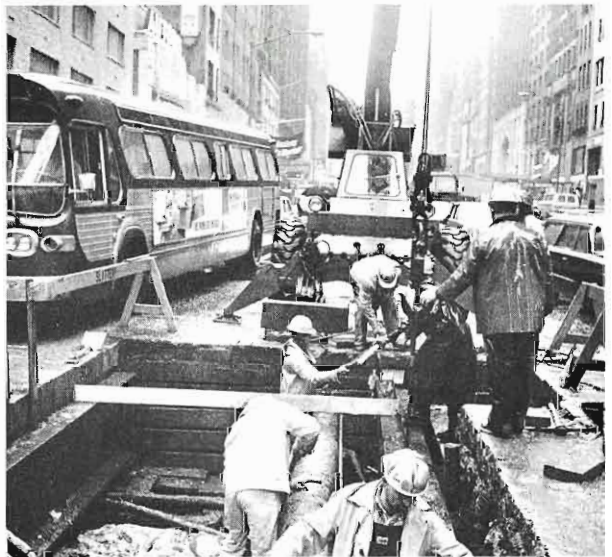
1964—construction in 57th Street
